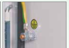
Protective ground connection Bolts on body and door
